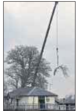
PLAN: A crane was brought in to remove the felled trees.
